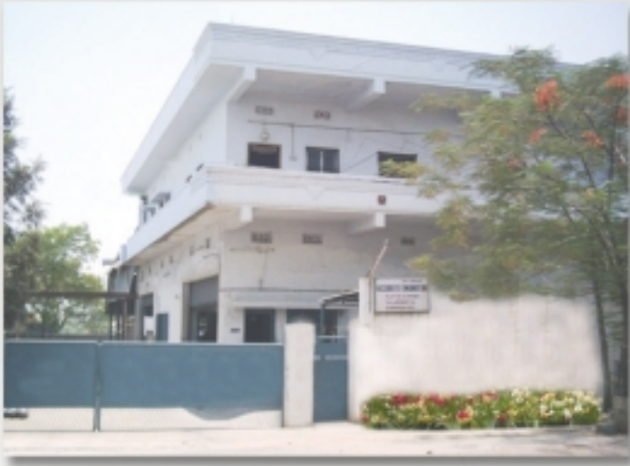
Our Factory Building
